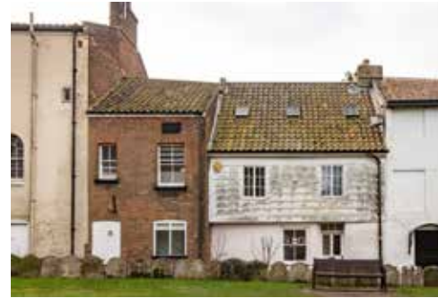
39 Market Place before (rear view)
